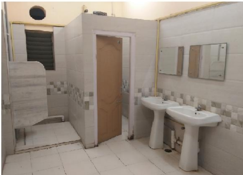
i) Photograph of some of the facilities
