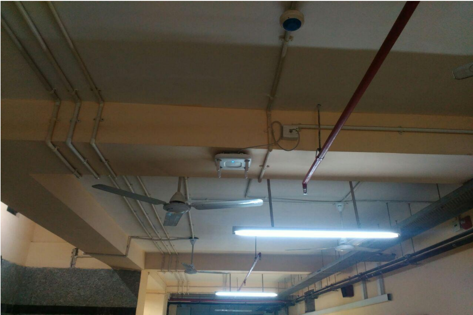
j) Photograph of Wifi Facility
